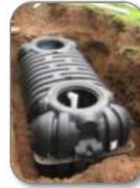
Flush: Septic tank
